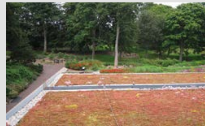
Extensively green roof—Botanic Gardens
