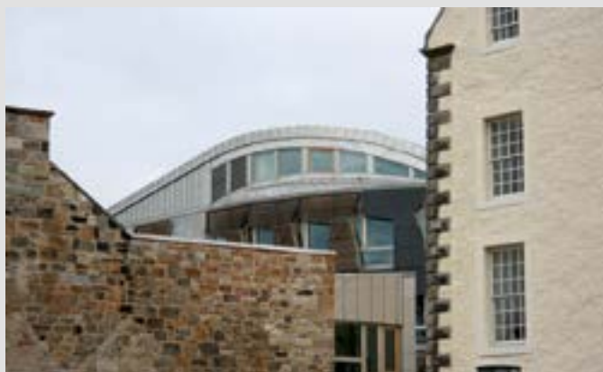
Metal roofing in a historic context—Canongate
