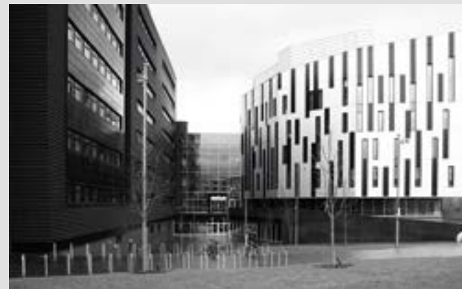
High quality detailing—Sighthill Court Construction of a sample panel and approval were required by condition in order to ensure the design intent of a high quality finish was executed.
