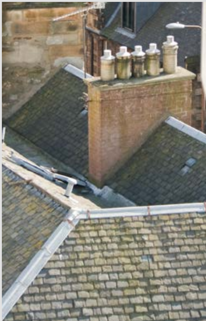
Traditional roofing materials (right)
