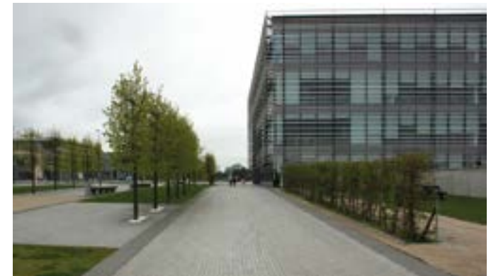
The office at Waterfront Avenue has a square in front and the space for a future public transport hub.
