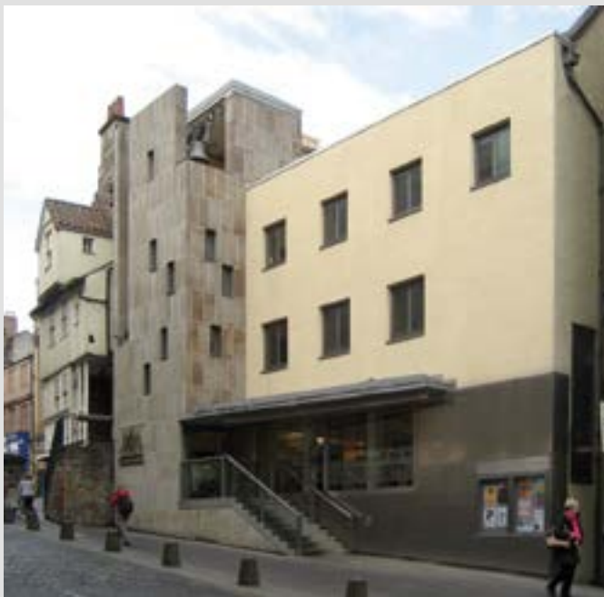
Integrating the new with the old—High Street
